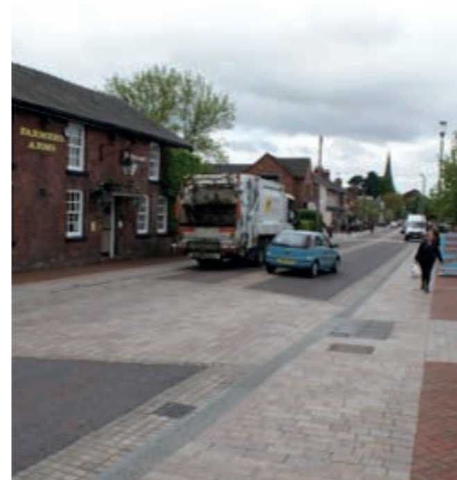
Figure 8: Narrowing of road carriageway, physically and visually
