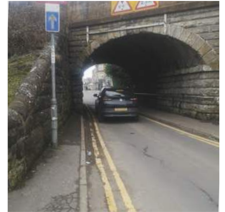
Springfield Road railway tunnel.
