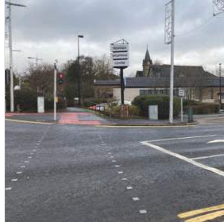
Existing pedestrian crossing at the Triangle Shopping Centre with library clock tower in background.
