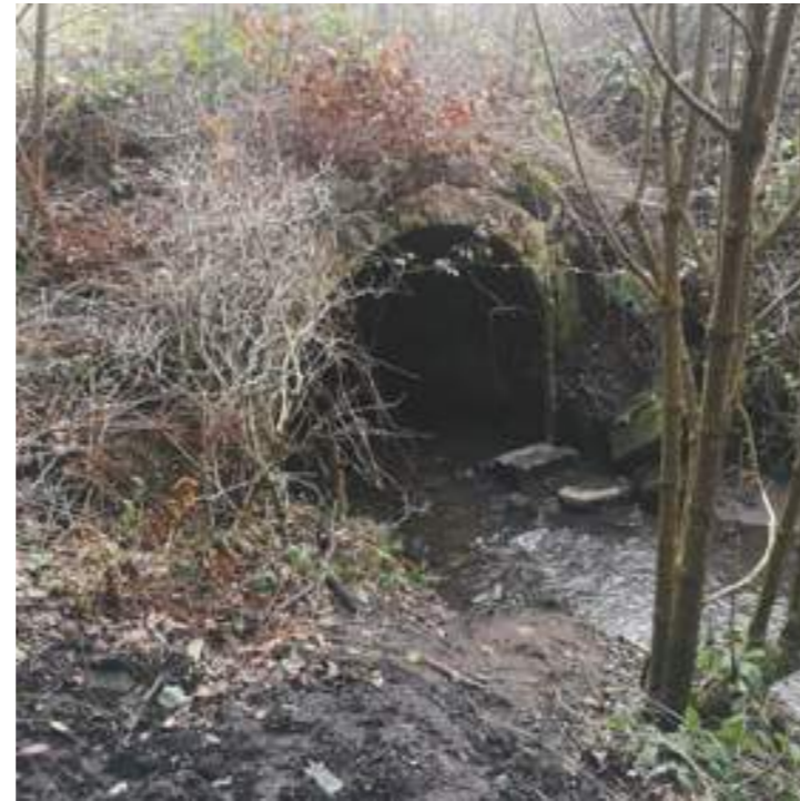
Exit from the Bishopbriggs Burn culvert into the park.
