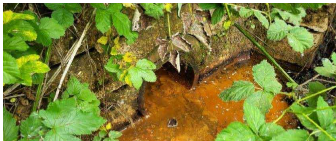
Plate 1 –ferruginous water (from the Aldi site?) entering the open ditch forming the south boundary of the development site and forming part of the South Catchment Outfall; refer bullet point 1 in item 18.
