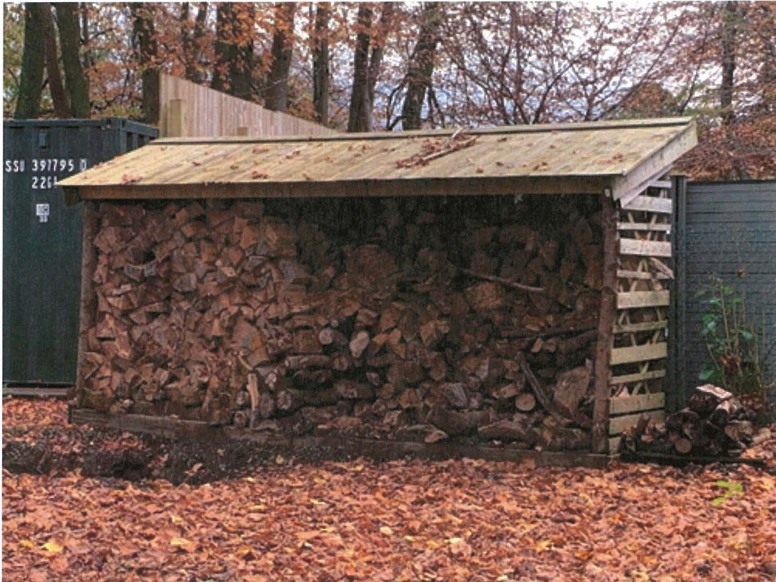
PHOTOGRAPH 2. The unauthorised erection of a log store structure.
