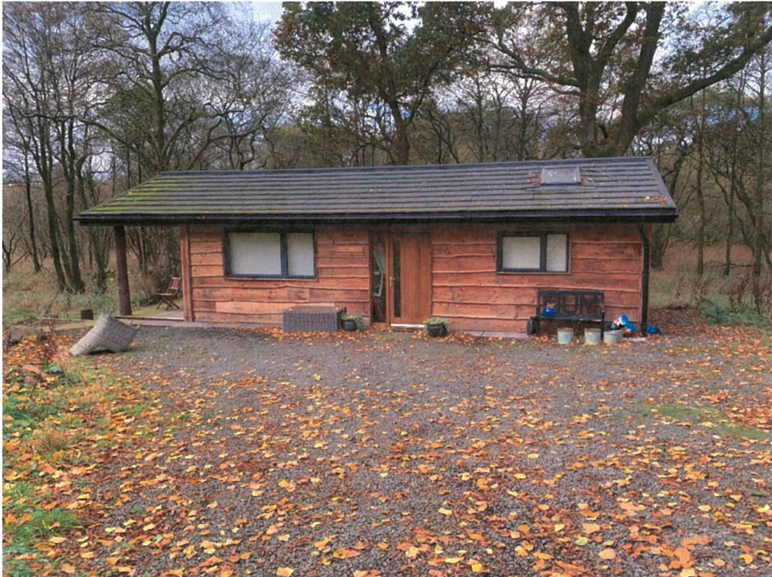
PHOTOGRAPH 1. The unauthorised erection of a single storey building (cabin) – “Bluebell Lodge”
