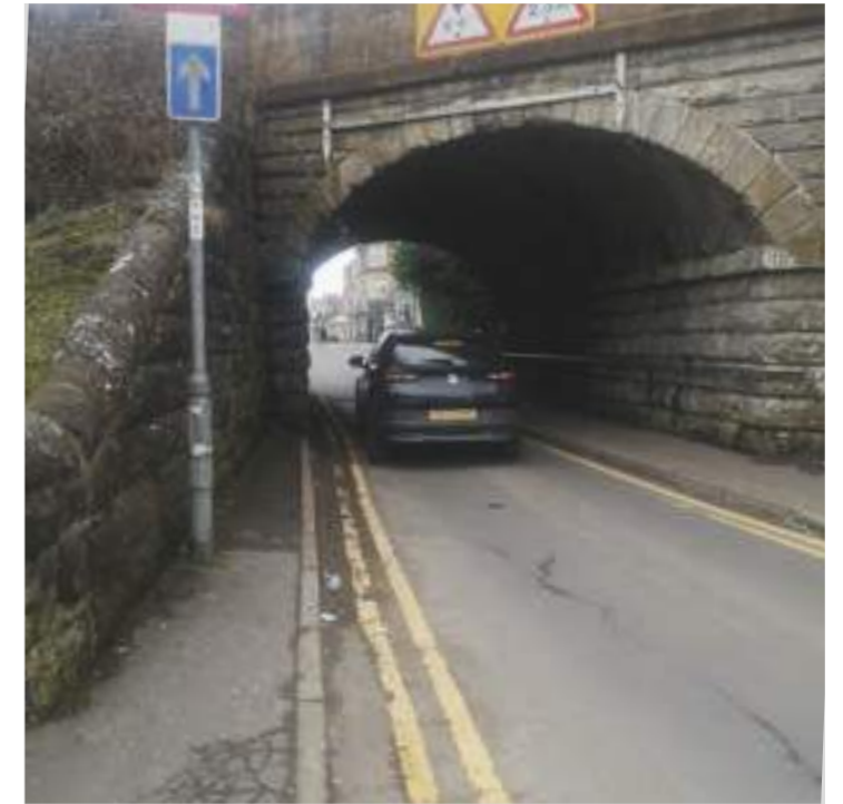
Springfield Road railway tunnel.
