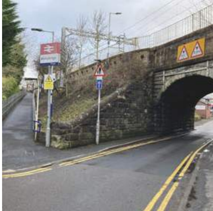
Access to the southbound rail platform from Springfield Road tunnel.
