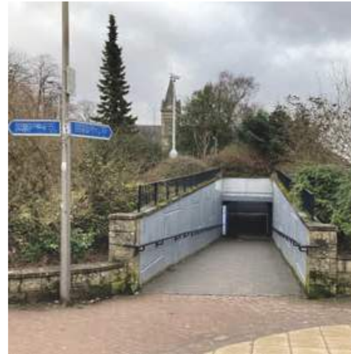
The A803 underpass from Bishopbriggs Park.
