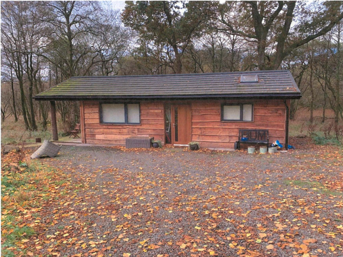
PHOTOGRAPH 1. The erection of a single storey building (cabin) – “Bluebell Lodge”
