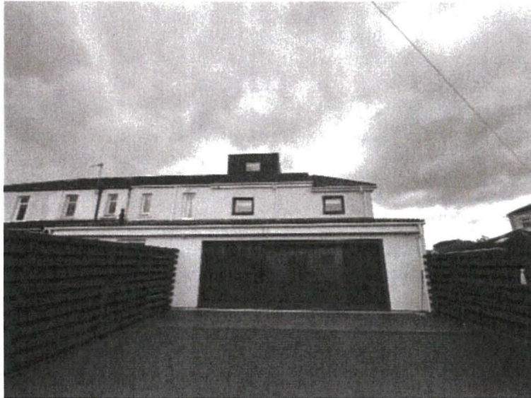
Image 2: Rear of property as built
