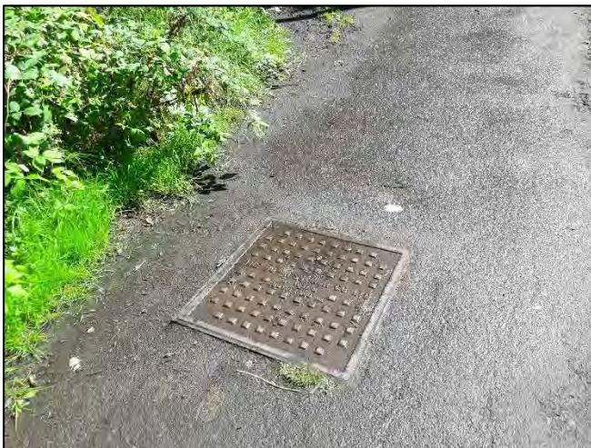
Manholes observed on public footpath
