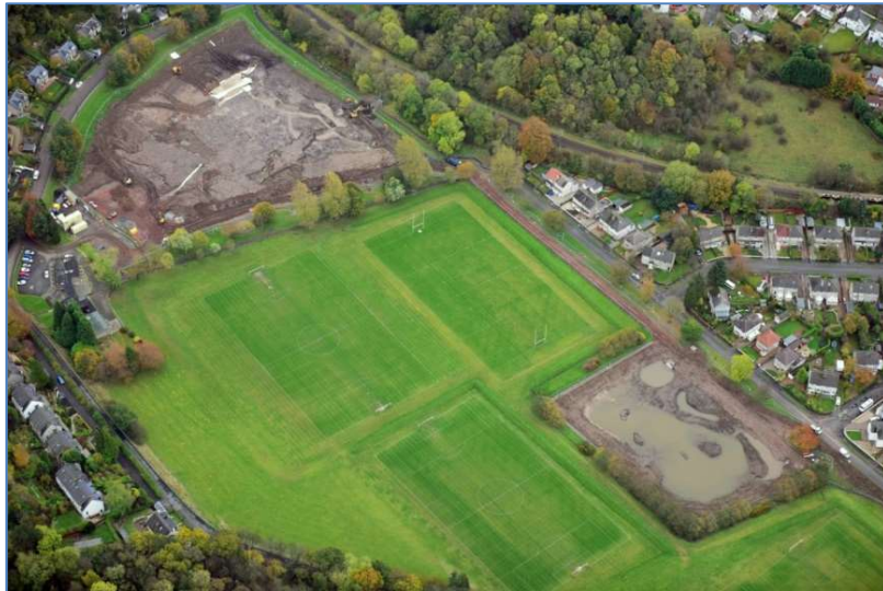
Work in progress: Construction of pond and wetland area, 2014
